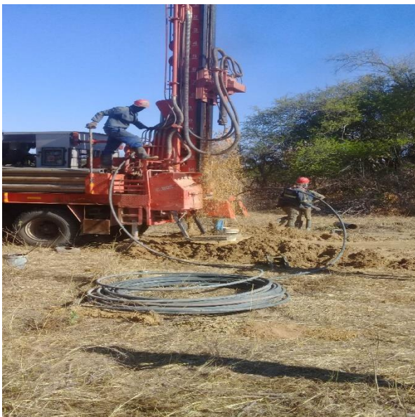
Figure 4 Borehole Drilling
