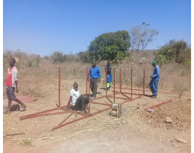
Figure 5 Fabrication of the 5 meter water tank stand
