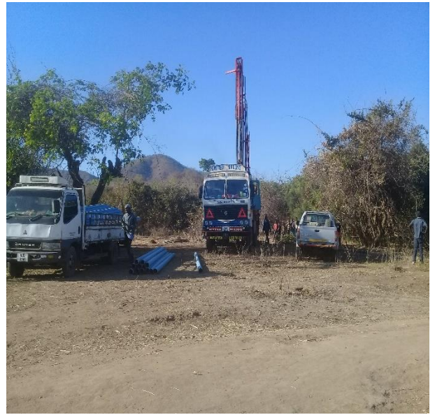
Figure 1 Drilling on the selected site
