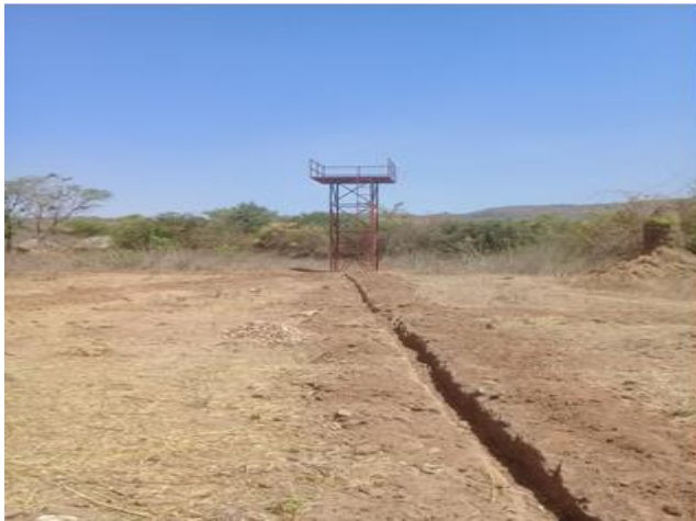
Figure 7 Preparing for laying of pipes
