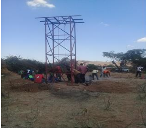
Figure 6 Erecting the water tank stand
