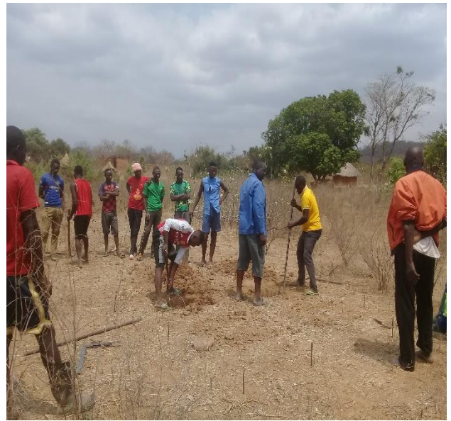
Figure 2 Digging a foundation for the Water Tank Stand
